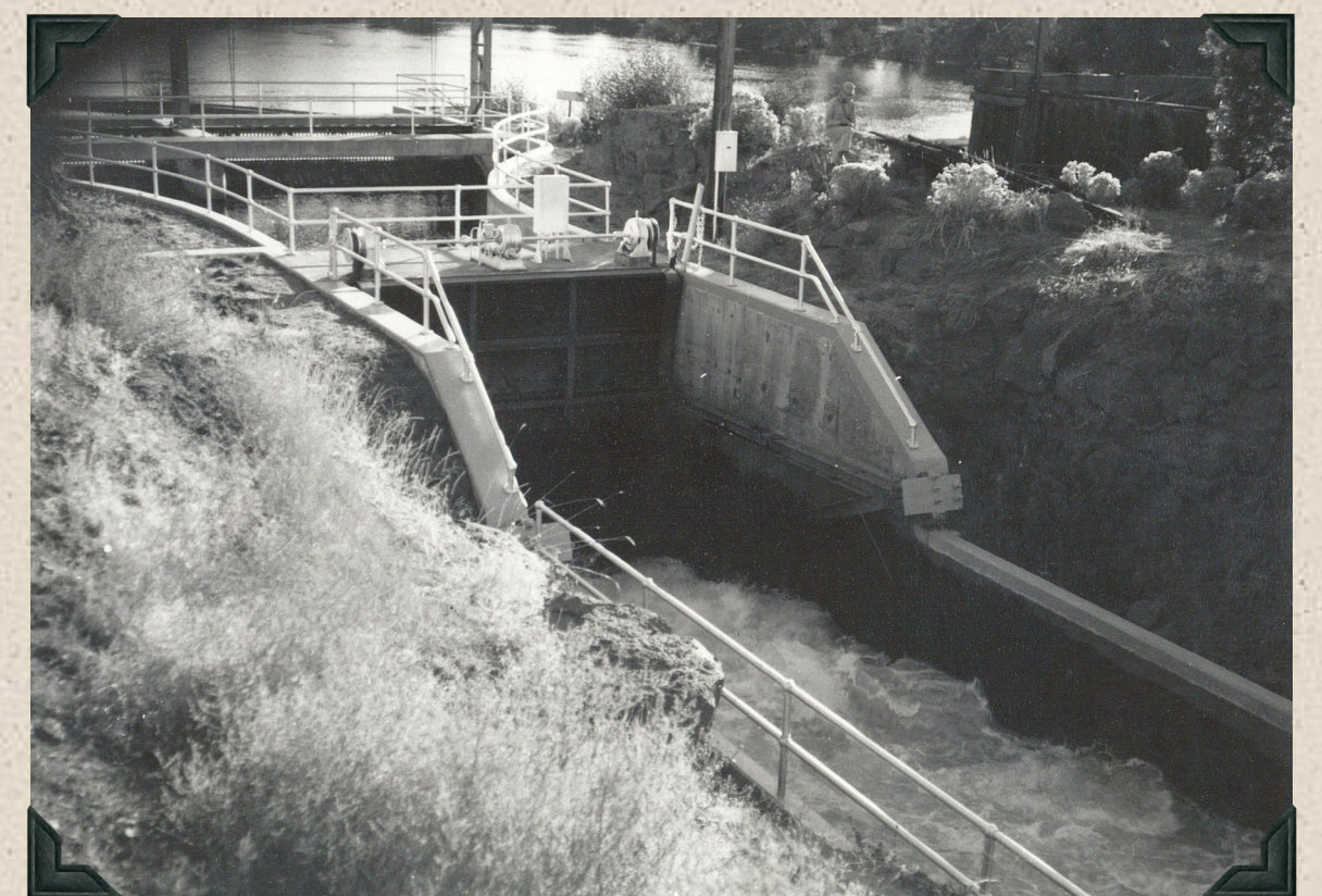
1952 - North Unit Main Canal Headworks Diversion gate structure for main canal.
