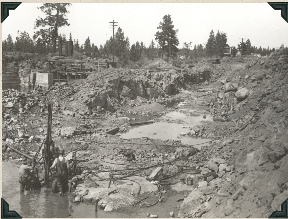
1941 - North Unit Main Canal Excavation for headworks.
