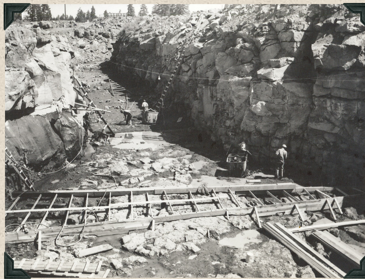
1941 - North Unit Main Canal Headworks Placing forms for headworks structure.
