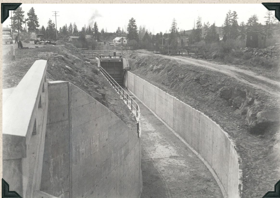
1942 - North Unit Main Canal. Looking upstream from the state highway bridge.
