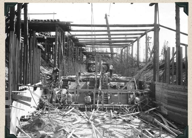
1940 - Wickiup Dam outlet works. Concrete finishing.
