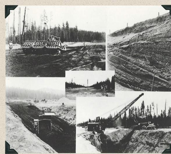
1939 - Wickiup Dam Embankment Civilian Conservation Corps (CCC) Top Left: Enrollees compacting fill on downstream face. Top Right: Type of soil excavated. Cut-off trench. Center: Stripping dam site. Bottom Left: Compacting cut-off trench. Bottom Right: Dragline excavating cut-off trench.
