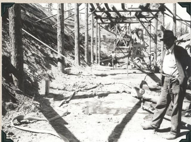
1940 - Wickiup Dam outlet works. Foundation grouting.
