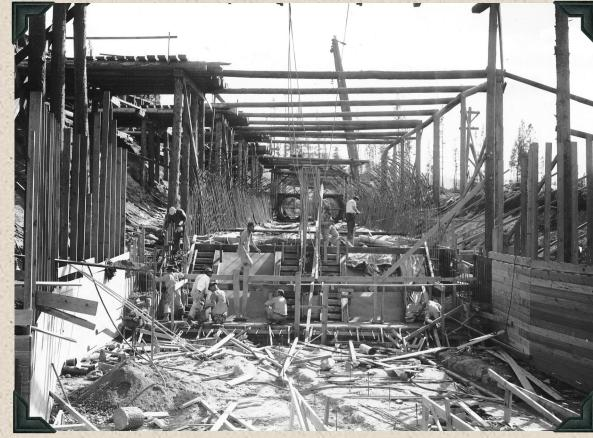
1940 - Wickiup Dam outlet works. Concrete finishing. Valve house structure.
