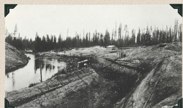
1939 - Wickiup Dam Outlet Works Top: Excavation and clearing begins. Bottom: Conduit excavation partially complete.
