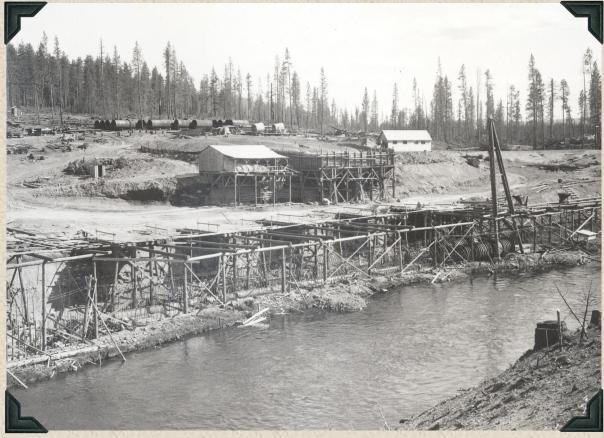
1940 - Wickiup Dam outlet works. Early stages of concrete construction.
