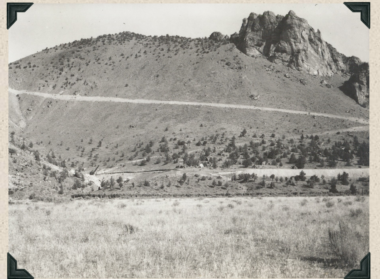
1941 - Road over Tunnel No. 1 (Burma Road) Sherwood Canyon.
