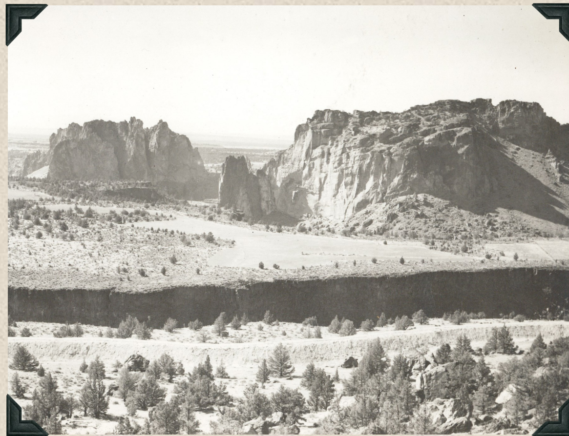
1941 - Smith Rock. North Unit Main Canal in foreground along the rim of Crooked River gorge.
