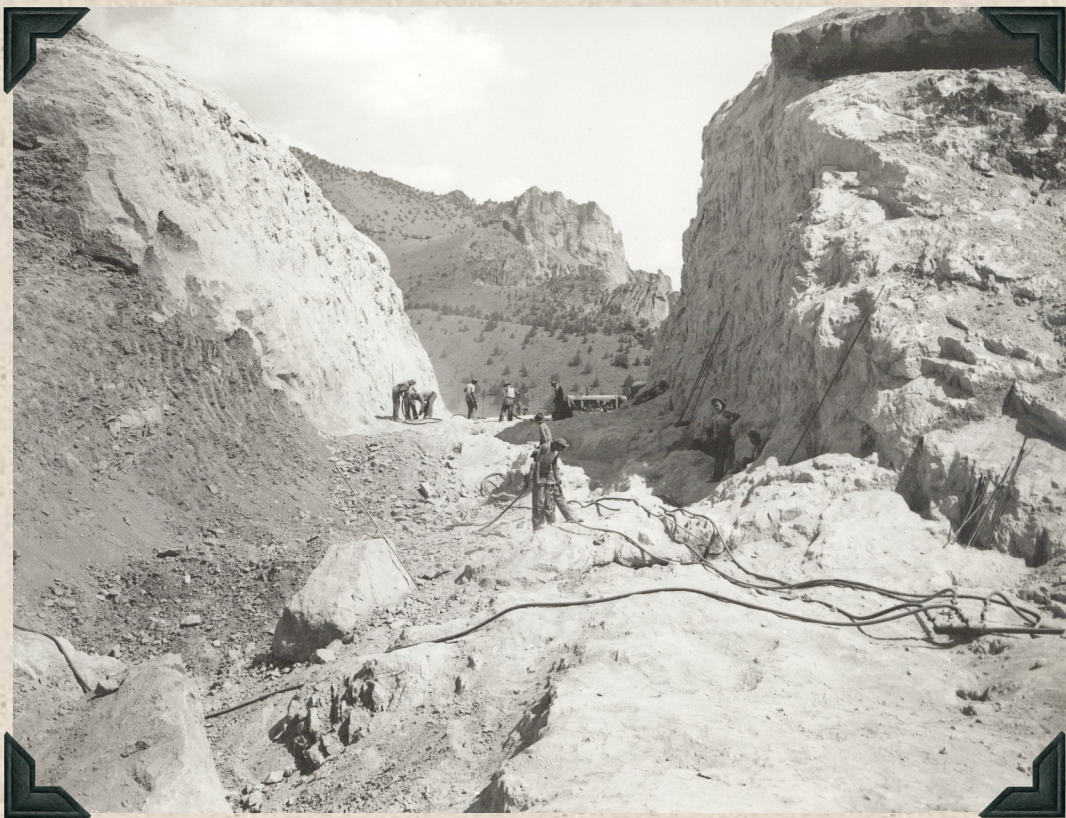
1941 - North Unit Main Canal. Drilling rock cut.
