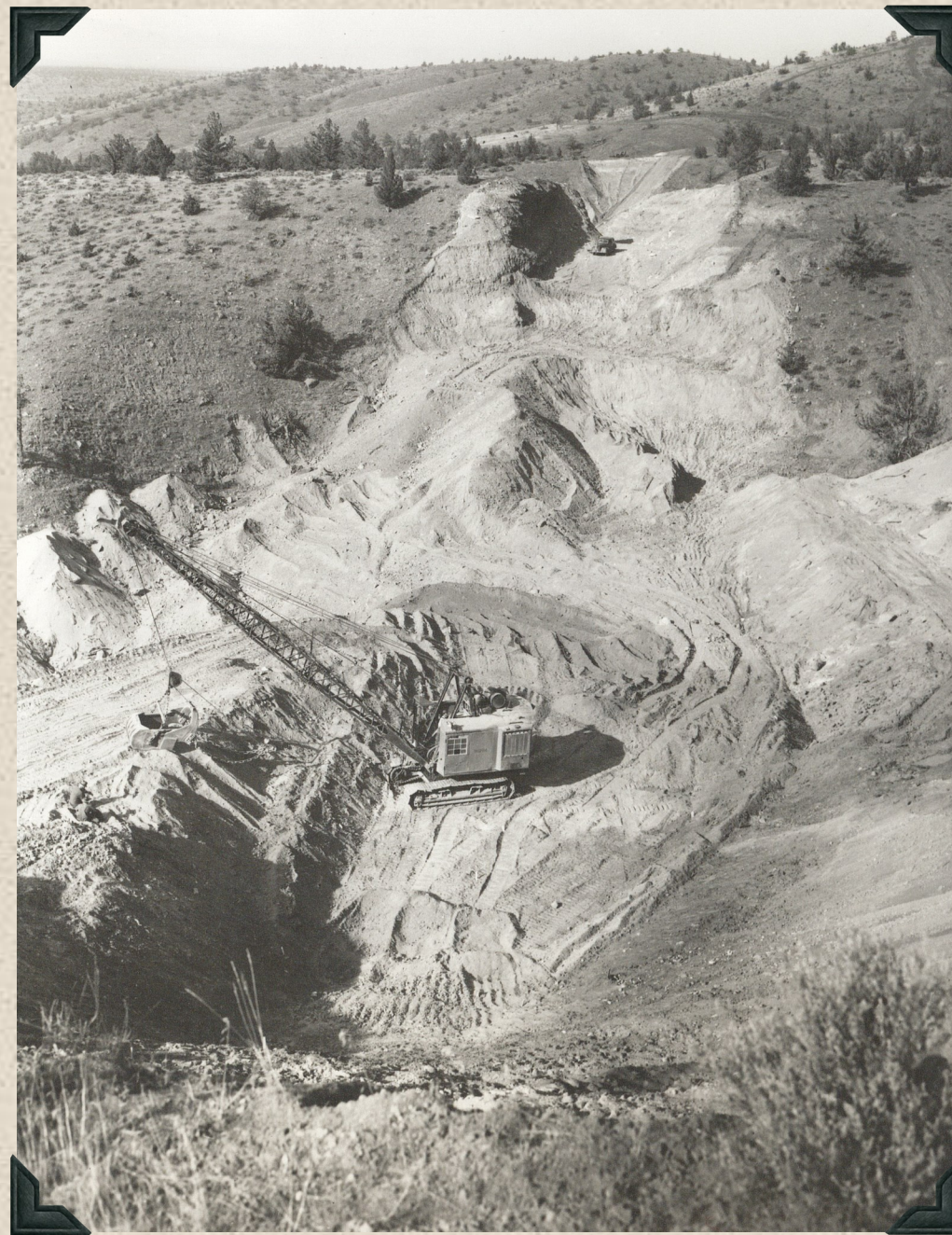
1941 - North Unit Main Canal. Excavating for outlet portal. Tunnel No. 2.
