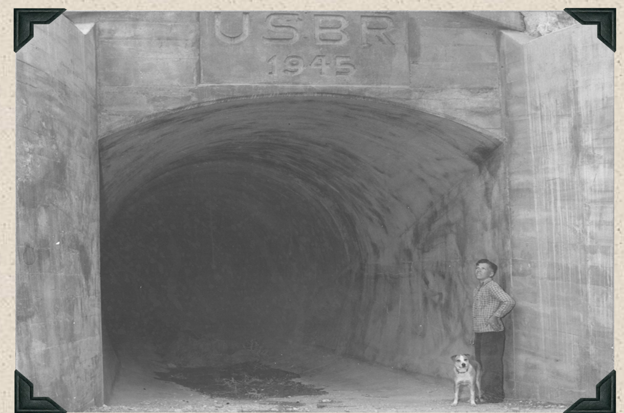
1945 - North Unit Main Canal Tunnel No. 1. Jackie Smith - 13, standing at the entrance to tunnel near Smith Rock.
