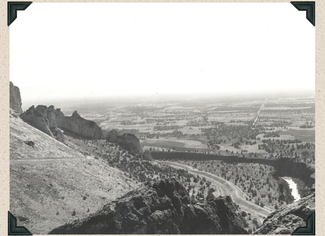
1941 - North Unit Main Canal. Looking south from summit of operating road over Tunnel No. 1. Crooked River Gorge in right foreground with finished canal immediately to its left.
