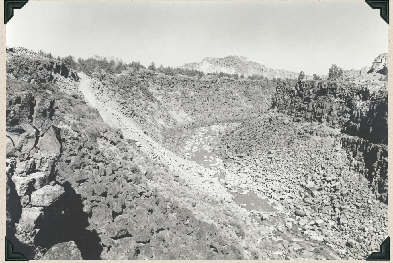
1944 - Site of Crooked River Crossing for the North Unit Main Canal.
