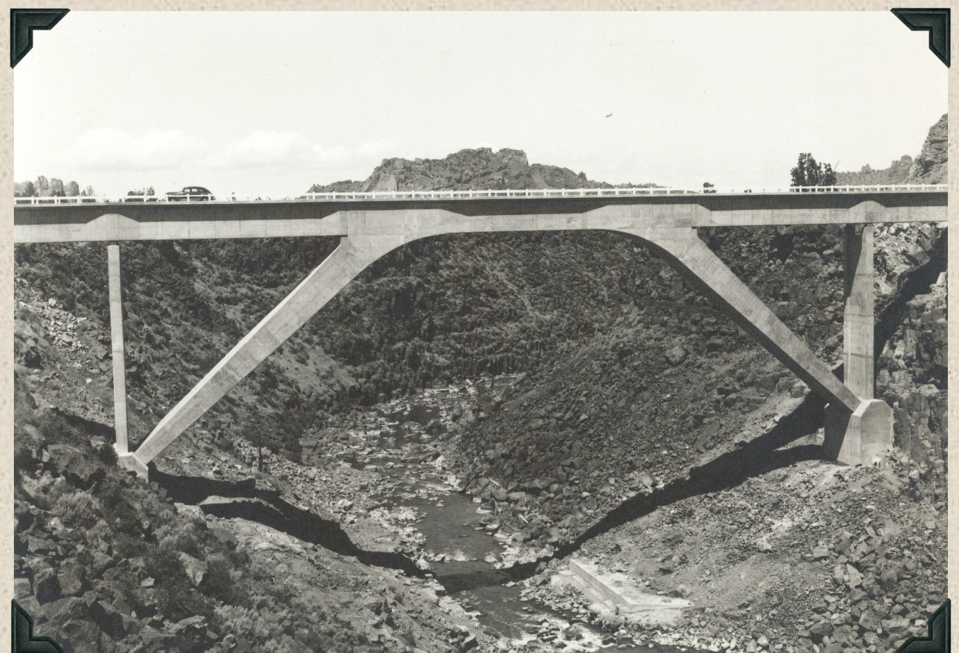
1946 - Crooked River Crossing, North Unit Main Canal. View of completed structure looking downstream from south rim of canyon.
