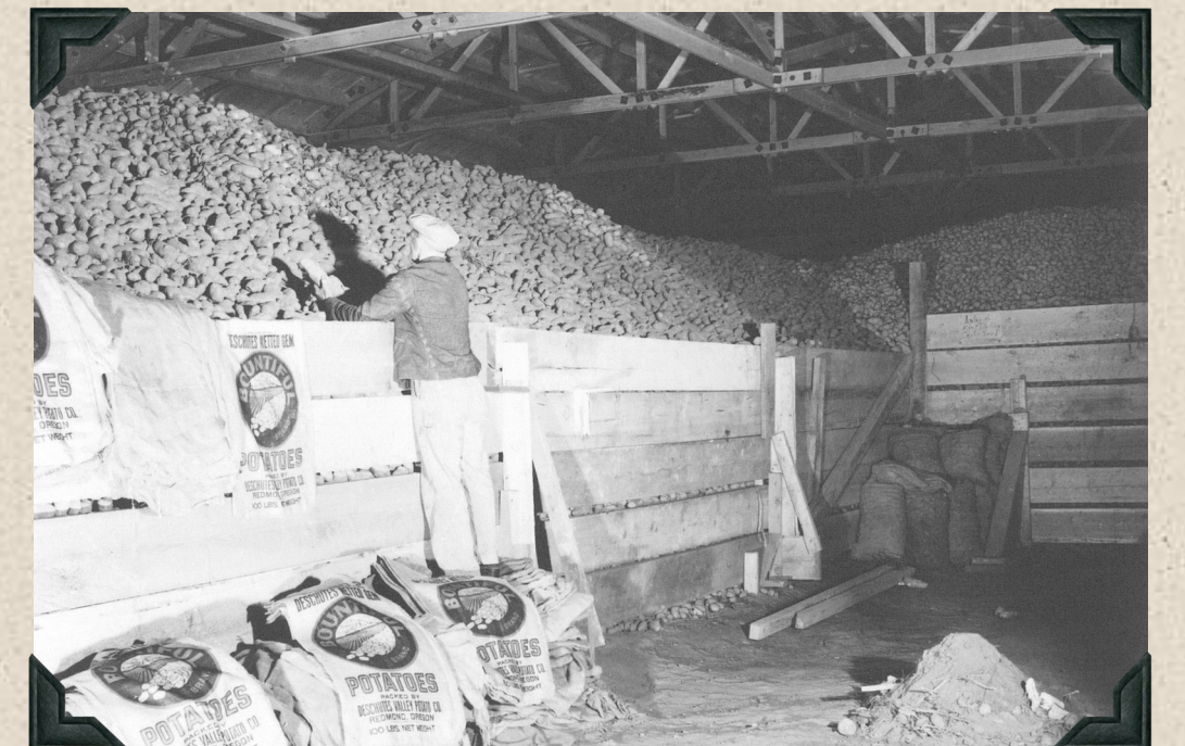
1947 - Deschutes Potato & Seed Co. Warehouse, Culver, OR. Checking a few of the 4,000 tons of potatoes stored, mostly certified seed for next year's planting.
