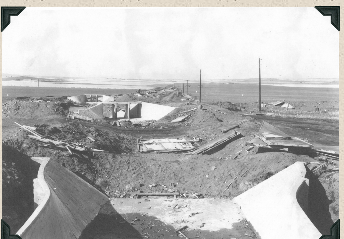
1946 - Looking downstream from foot plank of drop, Lateral M-43. Seven drops in view.
