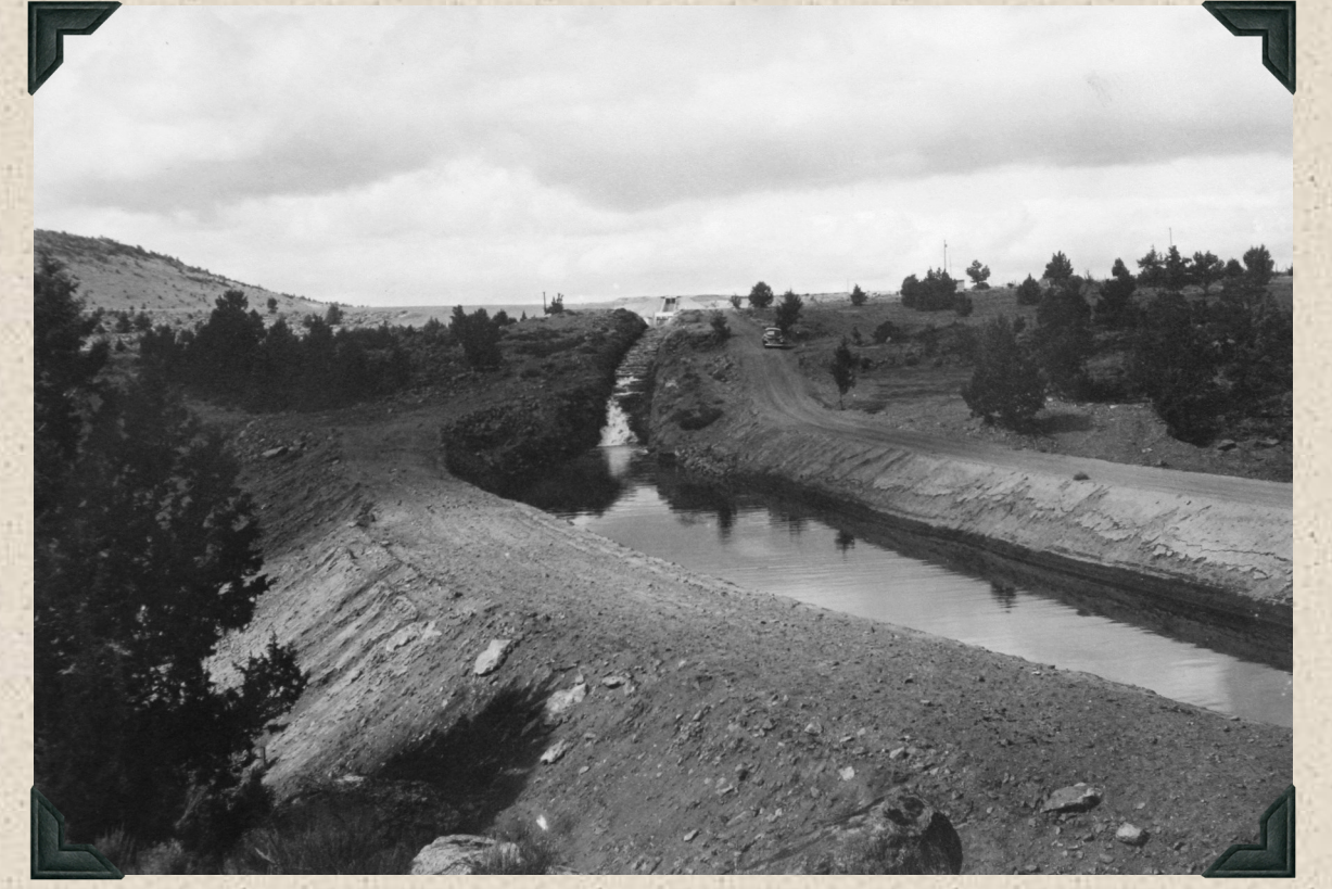
1947 - North Unit Main Canal. Prior to building Haystack Dam.
