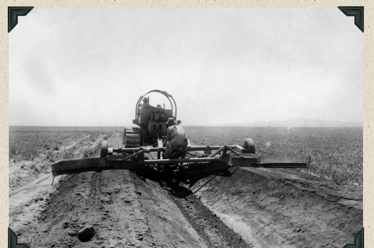
1948 - Rear view of Chattin Ditcher, Model 20-60, used by contractor, W.C. Bauman Co. on Agency Plains lateral system.
