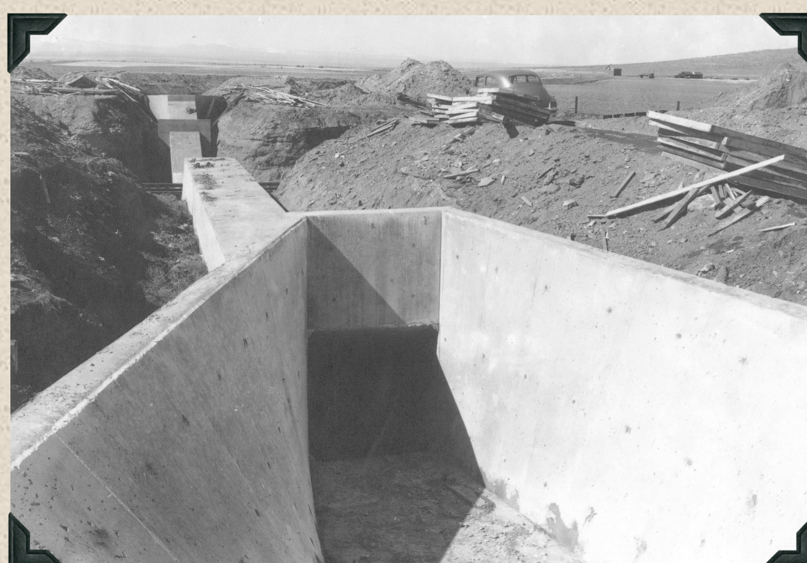
1946 - Highway and railroad crossing on Lateral M-43. Looking downstream.
