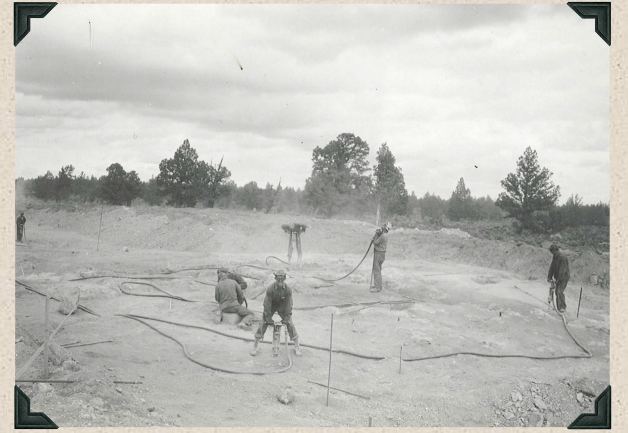
1940 - North Unit Main Canal. Enrollees drilling rock.
