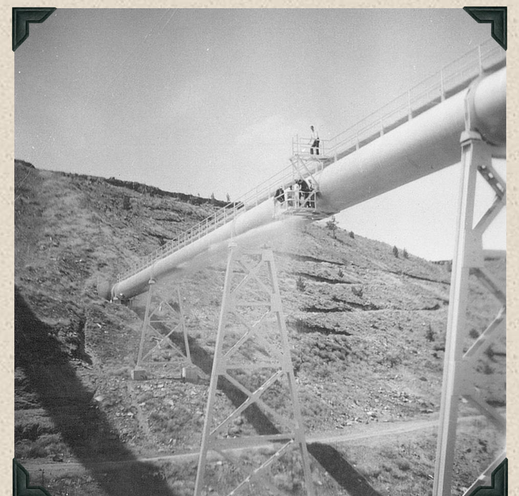
Willow Creek Siphon - Maintenance.
