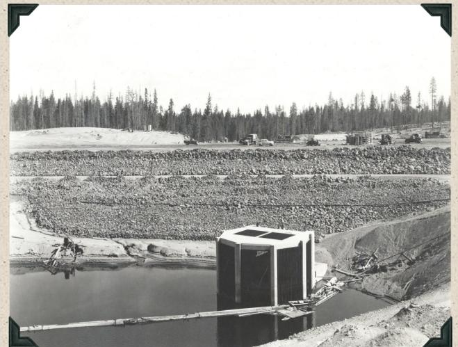
1942 — Wickiup Dam — Looking downstream from right bank. Trash rack structure in foreground, extension to hoist and gate chamber and top of valve house are in right background.
