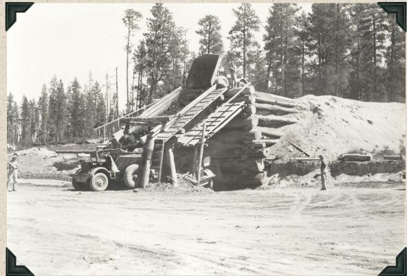
1943 — Wickiup Dam — Rebuilt grizzly used to segregate rocks. Material is dumped on inclined grate, rocks roll into dumpster at left and fines fall into truck underneath the grate.
