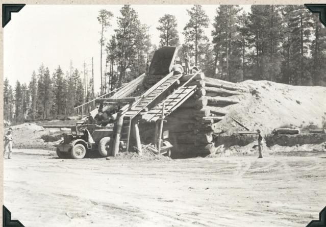
1943 — Wickiup Dam — Rebuilt grizzly used to segregate rocks. Material is dumped on inclined grate, rocks roll into dumpster at left and fines fall into truck underneath the grate.
