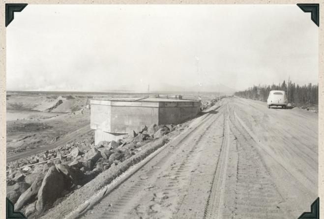
1943 — Wickiup Dam along axis. Nearly completed river section in foreground with control tower on left. Partially completed left abutment extending into background.
