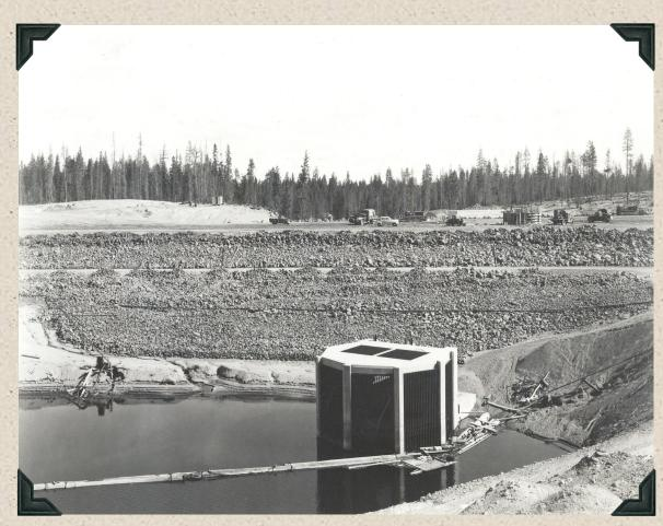
1942 — Wickiup Dam — Looking downstream from right bank. Trash rack structure in foreground, extension to hoist and gate chamber and top of valve house are in right background.
