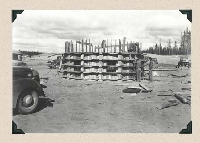
1942 — Wickiup Dam — Bureau forces placing forms for a six foot extension to the hoist and gate chamber. Extensions will be made in six foot lifts as work on the dam progresses.
