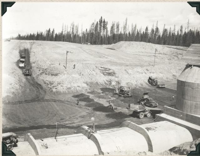
1941 — Wickiup Dam — Embankment placing in cutoff trench and river bed
